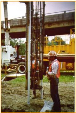
Figure A-4: 3' Diameter Test Drilled Shaft
