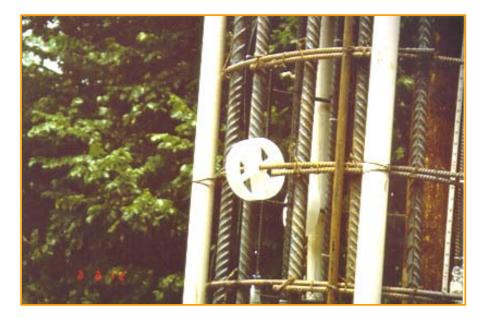
Figure A-10: Rebar Cage with Plastic Spacers attached to spiral reinforcing bars
