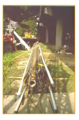
Figure A-3: 4-PVC CSL Access Tubes & 4" Steel Tremie pipe
